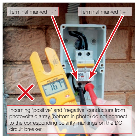
Polarity sensitive DC circuit breaker wired incorrectly
