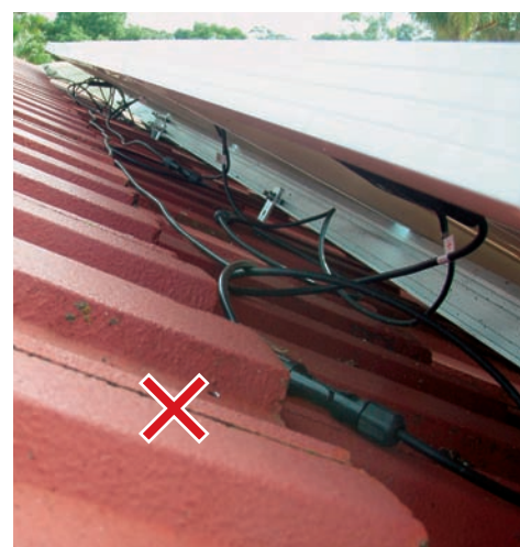
PV string wiring not fixed in position and laying of roof
